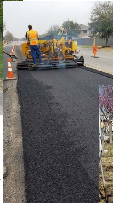
↓ Public Works Streets division installing a 2" layer of black base prior to repaving a section of Cibolo Valley Drive
