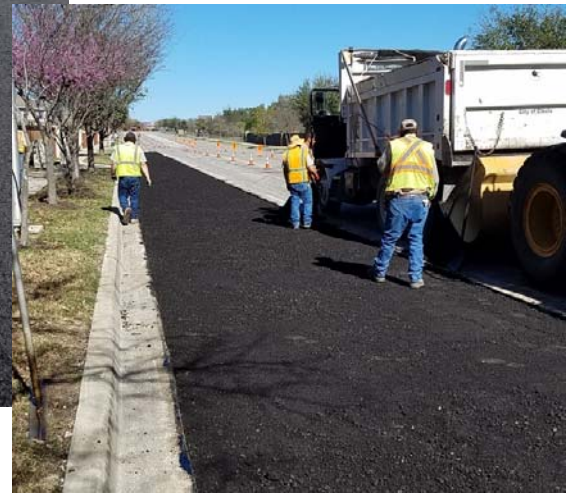
↓ Public Works Streets division installing a 2" layer of black base prior to repaving a section of Cibolo Valley Drive
